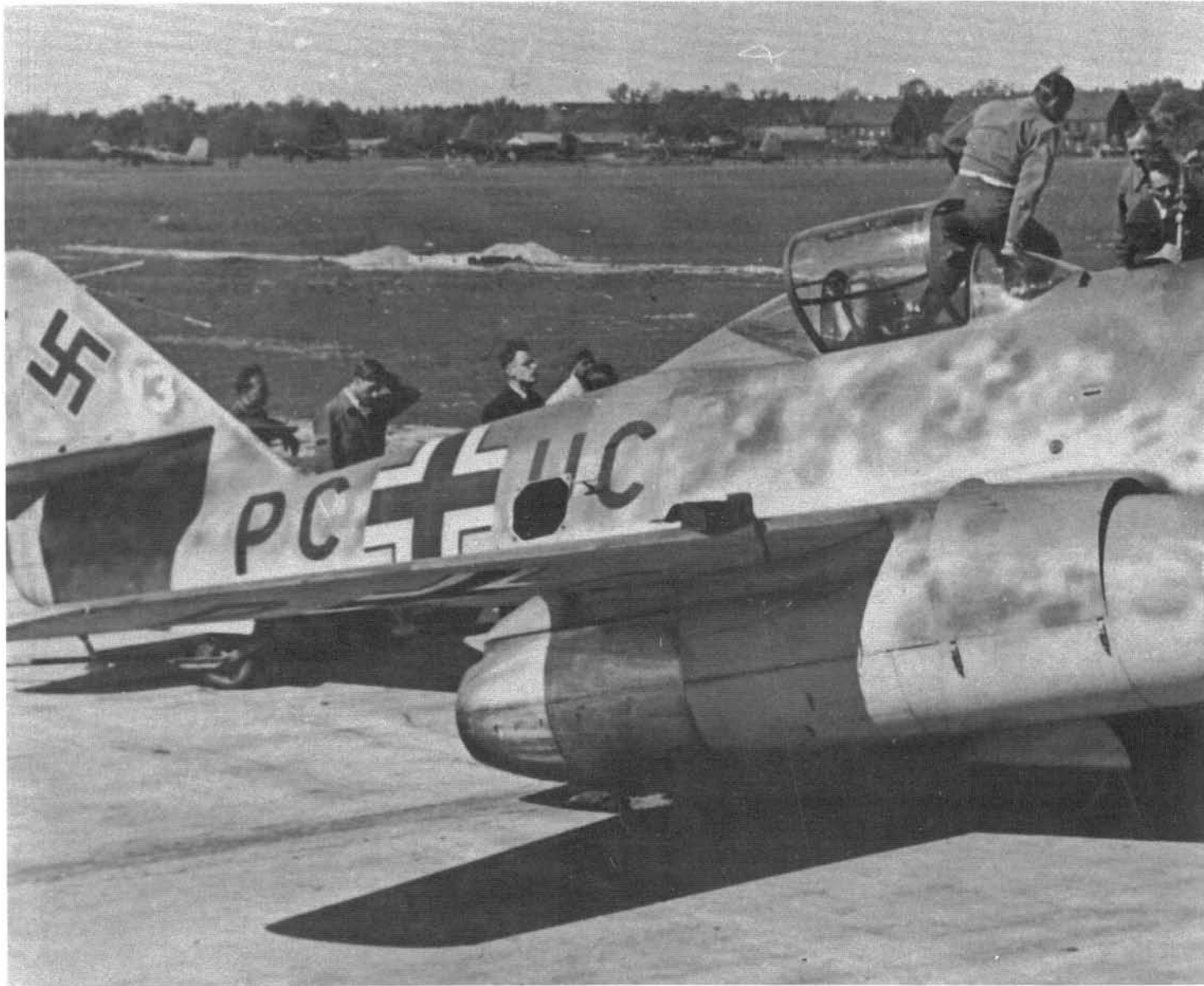
The Me 262 V3 at Lager Lechfeld: this aircraft's role in the test program was mainly high-speed trials and aerodynamic investigations (pressure distribution, the influence of Mach number, etc.). Note the He 177s in the background.
