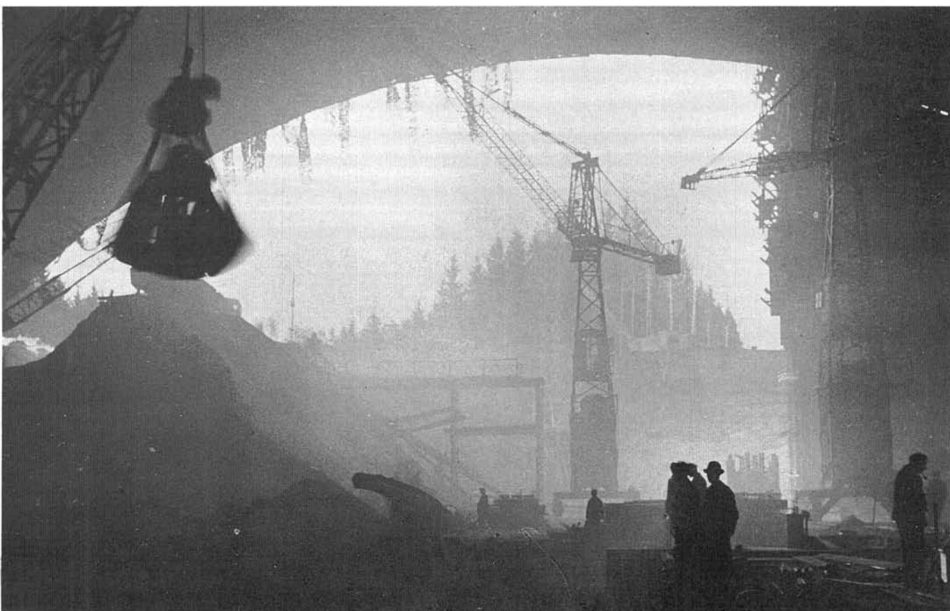
The concrete has set, the "core" of the first phase can be removed.
